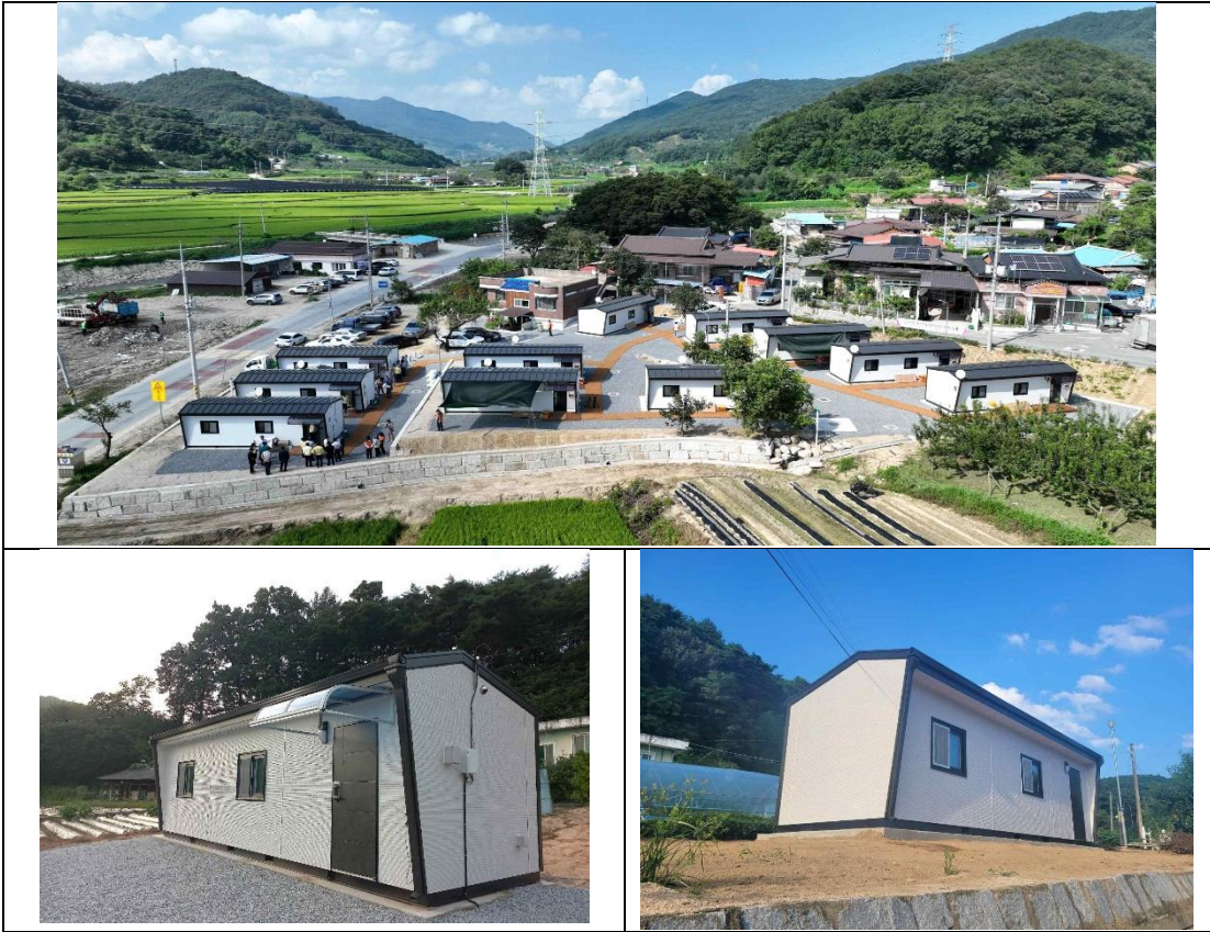
Figure I-4. Temporary houses for the victims of typhoon KHANUN and flood
